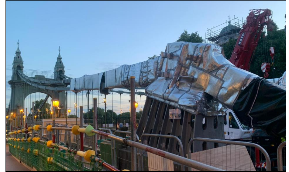
Photograph of Hammersmith Bridge pioneering cooling system during the summer 2023 heatwave, ensuring the bridge remained safe and operational. Source – Hammersmith & Fulham Council website
